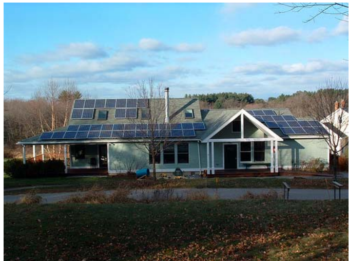
Solar Panels on the New View Common House in Acton
