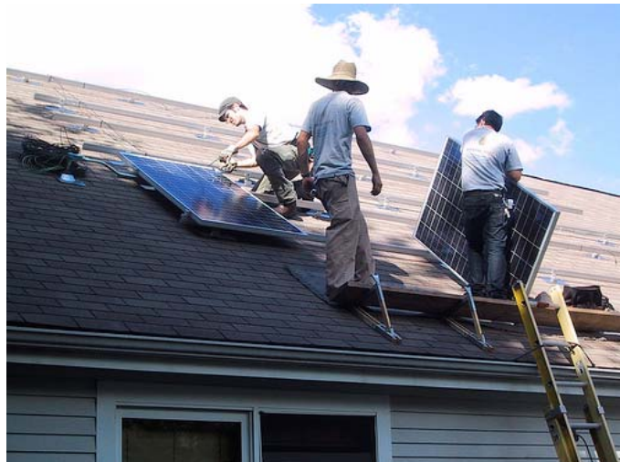
Panels at 18 Half Moon Hill - Going Up
